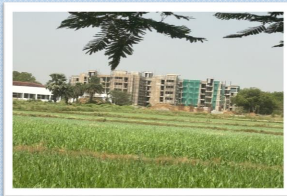
New hostel under construction
