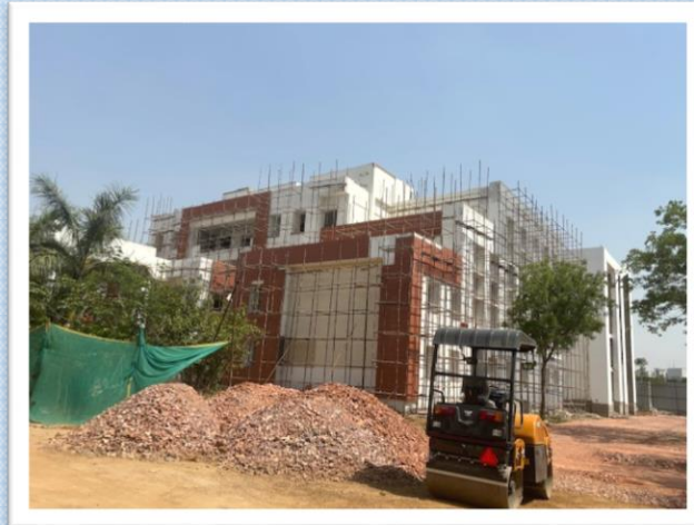
New academic building under construction in the Campus of SGIDT, Patna.
