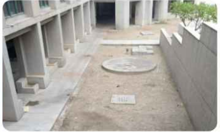
Rain Water Harvesting (16 units)
