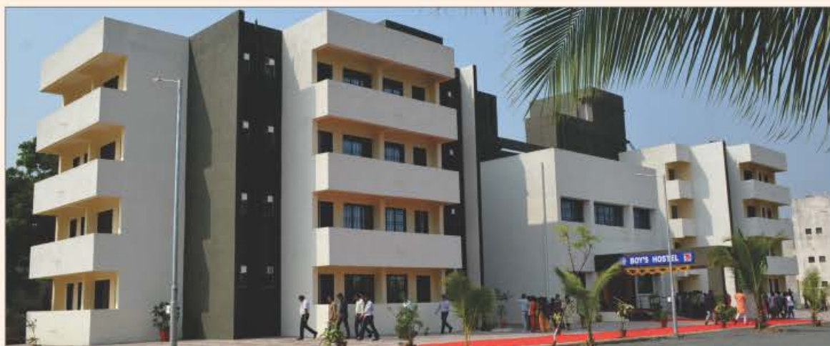
Construction of Boys Hostel is Completed. Grant received from RUSA.
