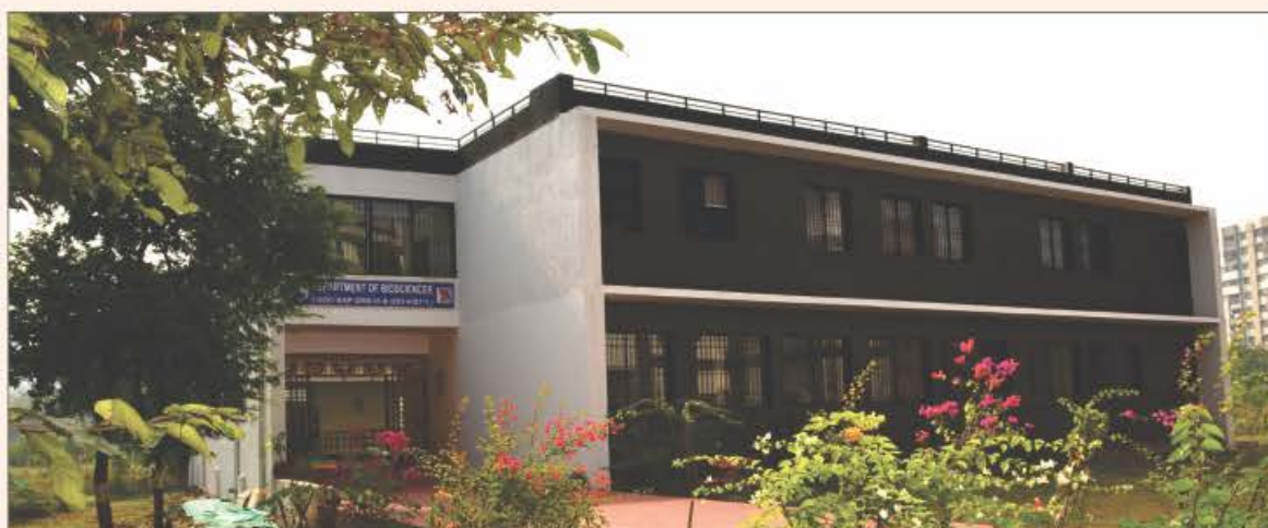
Construction of Laboratory for Bio Science Department completed. Grant received from RUSA.
