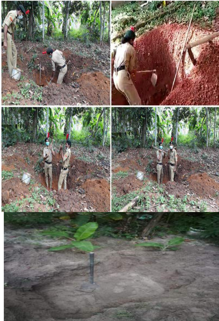
Rain Water Harvesting- digging pits for collecting rainwater in the campus premises
