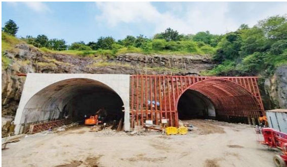
Tunnel entry and exit points under completion
