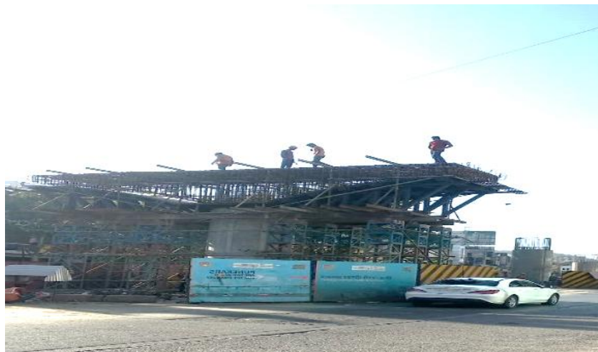
Figure 2: Flyover Construction at Research Site
