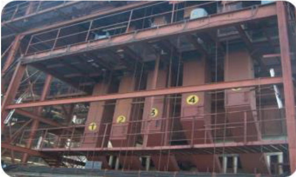
Bagasse Silos & Feeders of Boiler
