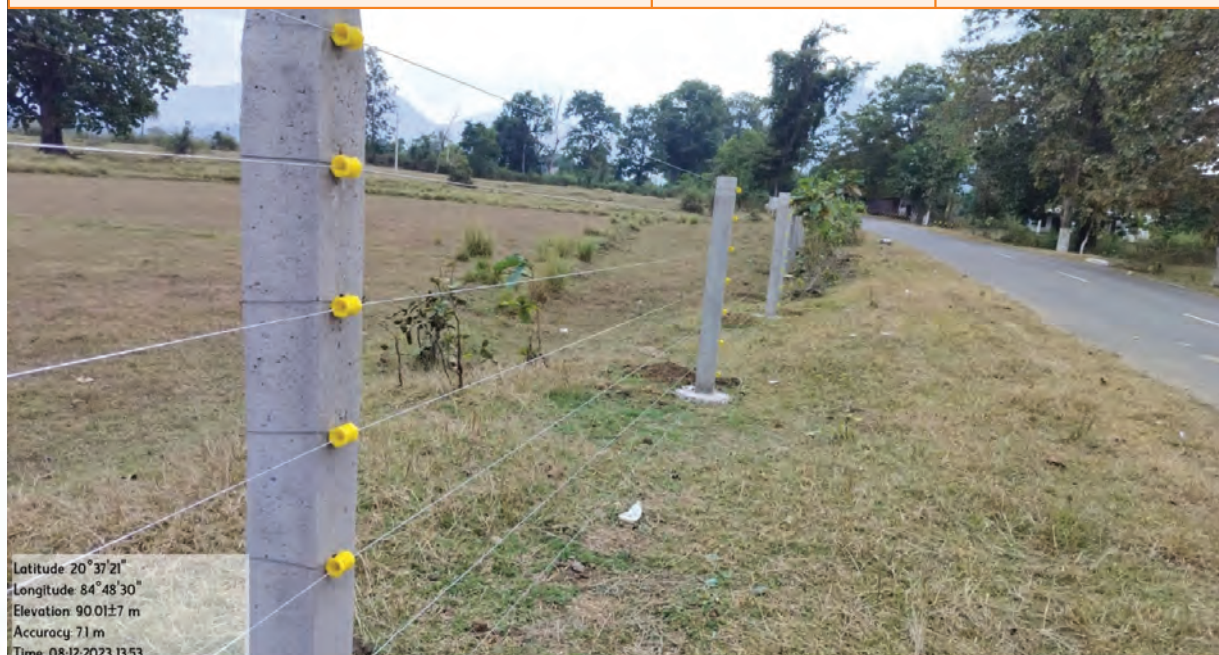
Solar Fencing work at Hatibari under Satkosia Wildlife Division
